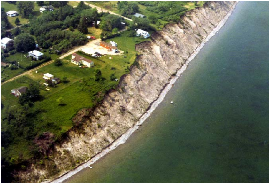
Erosion of high bluffs along the south shore of Lake Ontario
